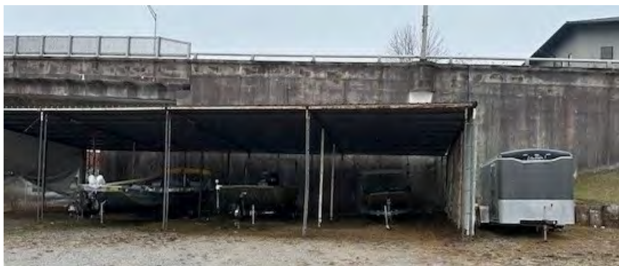
Figure 5.1 BGE Boat and Trailer Storage
