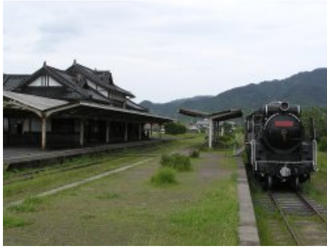
Figure 5-1: Abandoned railroad and station, near Taisha (Shimane Prefecture) The landscapes of depopulated areas are often full of abandoned buildings such as this railroad and train station.
