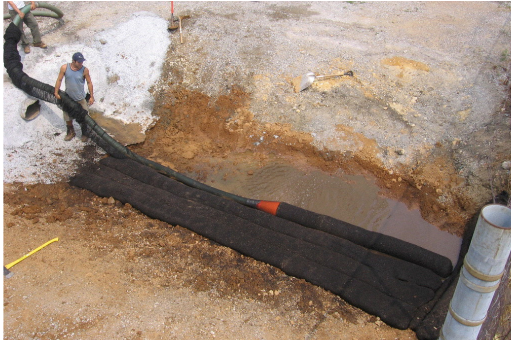
Figure 1: Installation of Filtrexx SOXX at the Chattanooga Parking Facilities
