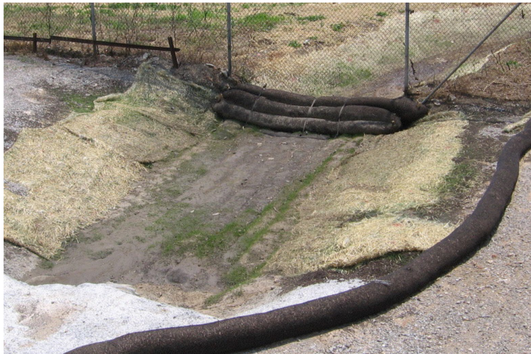
Figure 2: Two weeks after installation
