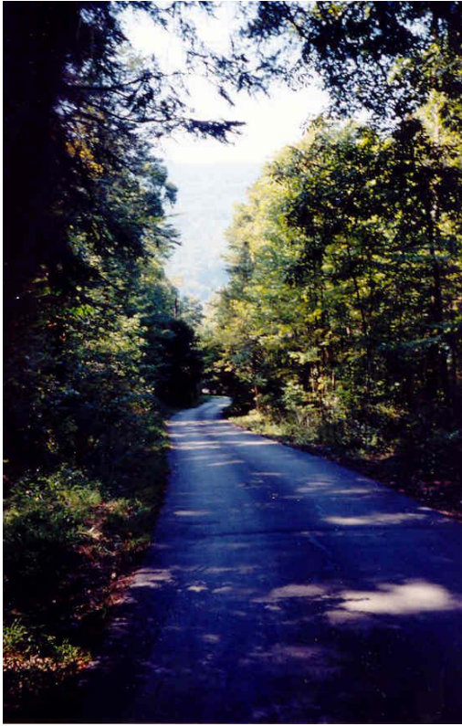
Looking down the main driveway.
